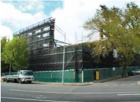
EXTERNAL SOUTH-WEST CORNER, DEMOLITION STILL UNDERWAY, APRIL 2010
